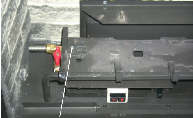
Secure burner to valve tray.
